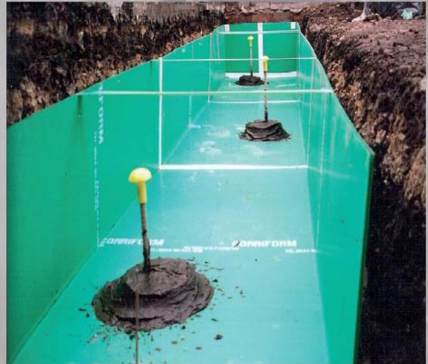
Shuttered trench ready for Tencon Concrete pour.
